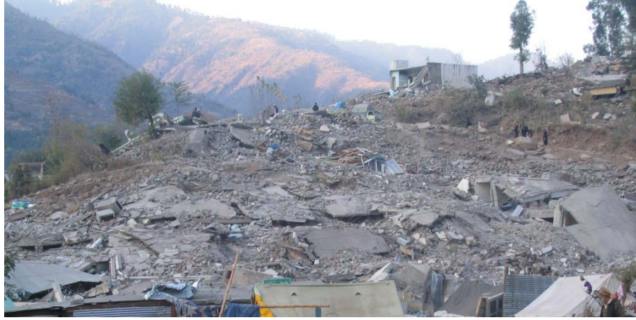
Damage in NW Balakot (T.Rossetto, UCL/EEFIT).
